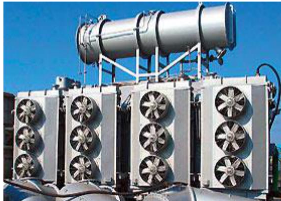
Trafo 400 MVA, EMS – TS Obrenovac
