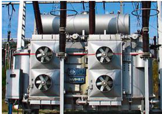
Trafo 150 MVA, EMS – TS Jajinci
